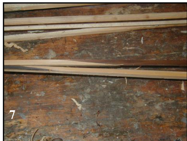
Photo 6 shows gluing the scarf. Photo 7 shows a glued scarf.
